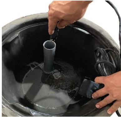
Pass the cord from the pump down the cord pipe and retrieve it at the base.
