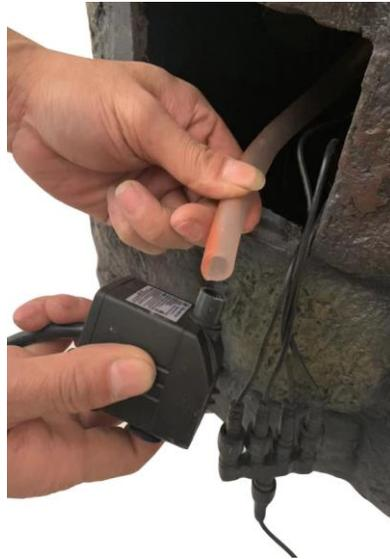
Locate the pre-installed tubing and attach it to the pump.
