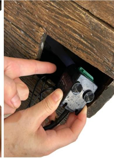
Place the pump with tubing attached inside the fountain body.
