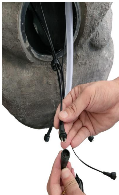
Using the threaded connector, securely attach the lights to the connections from the pump.
